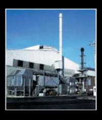
The HF dry sorption system is equipped with several layers of honeycomb lime modules featuring a low pressure loss. The Ca(OH)<sub>2</sub> modules react with the hydrofluoric acid contained in the exhaust air and calcium fluoride(CaF<sub>2</sub>) is produced as end product.
